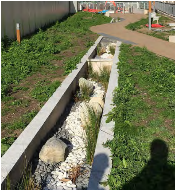
SUDS water channel (construction prototype)
