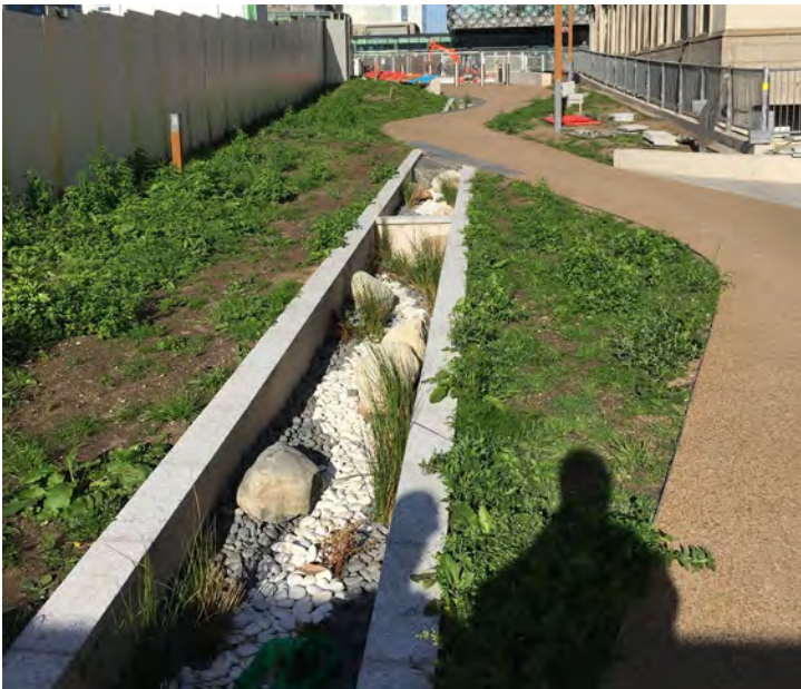
In-Construction - SUDS Channel (part of 2AC works)
